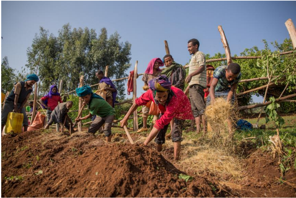
Ethiopia – digging trenches for water pipes
